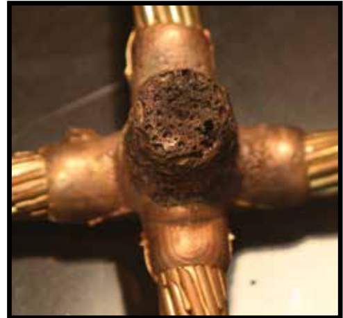
Image 6: Contaminated weld. Cables excessively dirty or moisture present.
